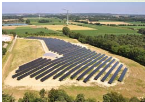
An open space system near Flamschen planned and built by Solen Energy
